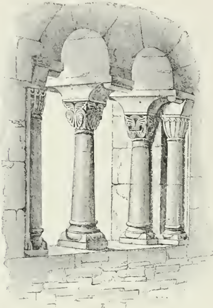
MIDWALL SHAFT: WINDOW IN CHURCH OF GERNRODE, GERMANY.
